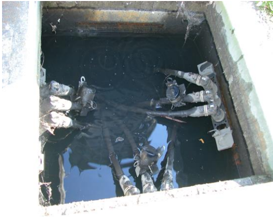
Figure 7-4: Load-Break Connections, Below Grade, Current Conditions
