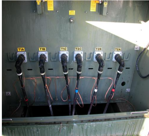
Figure 7-5: Load-Break Connections, Above Grade, Future Conditions
